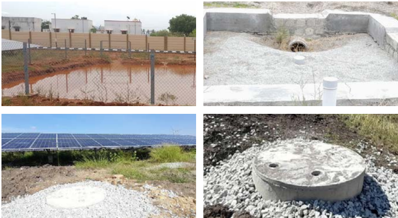
Artificial Recharge Pit constructed at WHS Power Project, Jagaluru, Karnataka & Dindigul Project, 58MWp
